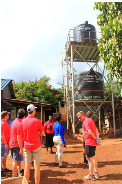
Water tank donated by St Edward's
